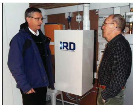
One of IRD's hydrogen-fuelled 1.5-kWAC and 1.5-kWth \mu CHP units installed in a Danish household.
